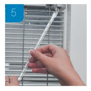
First, manually tilt your blinds to an open position (this is important for the configuration step later) and then remove the wand.
